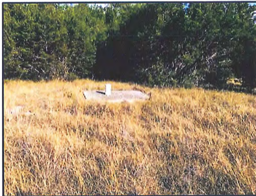
View of drilled water well in the southeast/central portion. The well is not equipped with a pump or electricity. Rancho Sierra includes several "test wells" which were drilled to ascertain water availability on the ranch.
